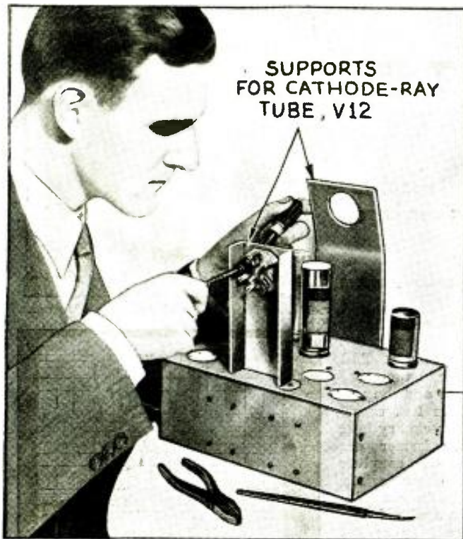
Fig. H. The C.R. chassis is the stages of construction.
